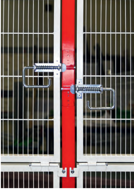
Upper folding field with maintenance opening and lock
